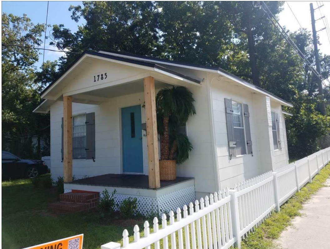
Existing building on site
